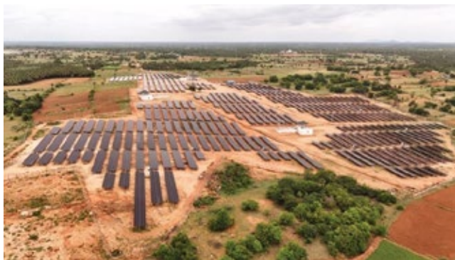
Open Access Solar
